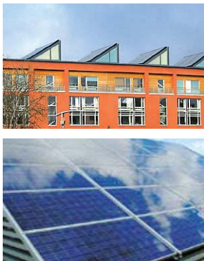
지붕 Solar Panels & Solar cells
